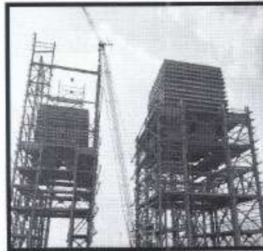
SILO construction progress
