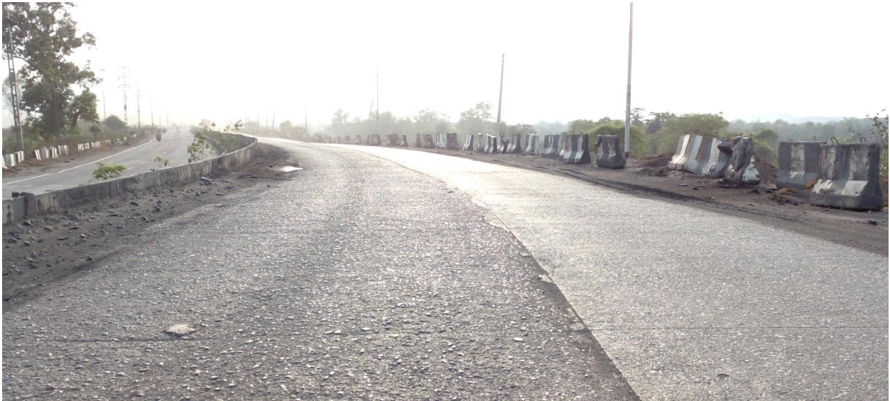
Concrete road of length 2700m and width 12m from Bankibahal towards Raigarh for HMV
