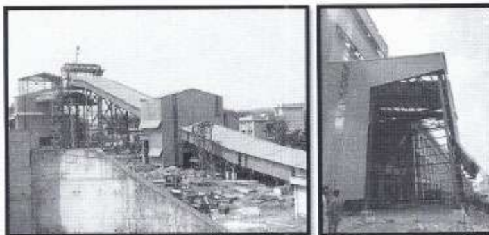
View from truck receiving hoppers routing to ground bunkers.
